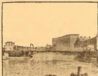
Constructed Dearborn Street Bridge, 1,450 Tons. —1907—
